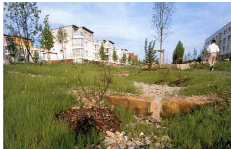
EXAMPLE - The restructured swale will mimic the broad character of the existing drain, yet will improve flow as a result of site ground levels and significantly increase filtration and water-holding capacity with deep filter beds. The swale will be designed in layers for capture and attenuation during high rainfall events. (UK).
