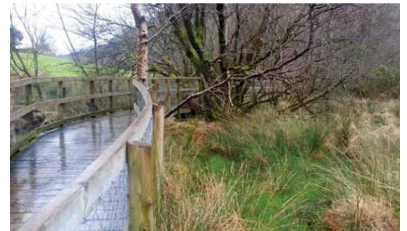
EXAMPLE - An elevated footpath can pass through the damp woodland with minimal impact on the habitat. Users come face to face with the internal workings of an otherwise inaccessible environment. (Glendalough, Co. Wicklow).
